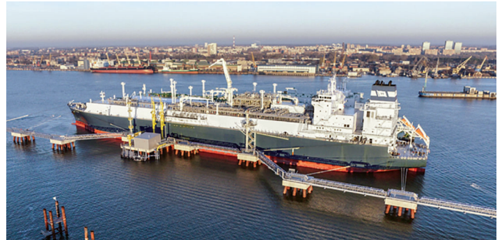
Poland has taken delivery of its first cargo delivered to Klaipeda FSRU
