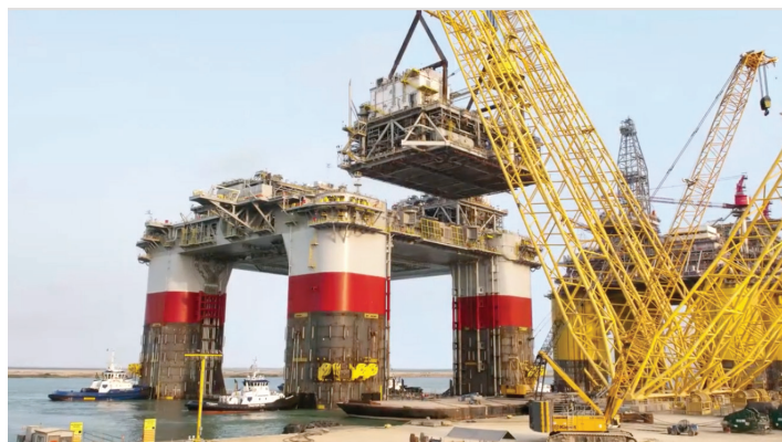
FLNG units to be built at Kiewit Offshore yard in Texas
