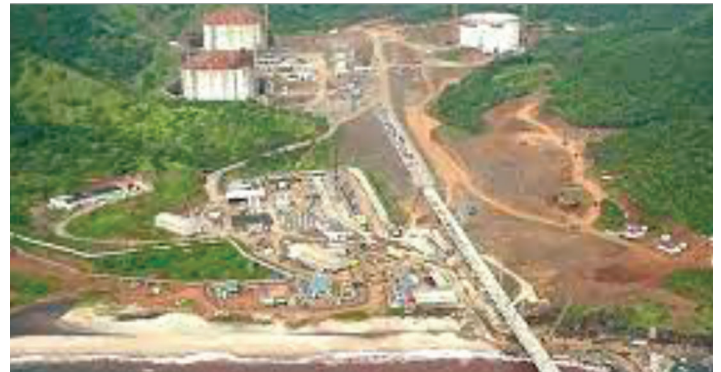
Dabhol LNG import terminal located south of Mumbai
