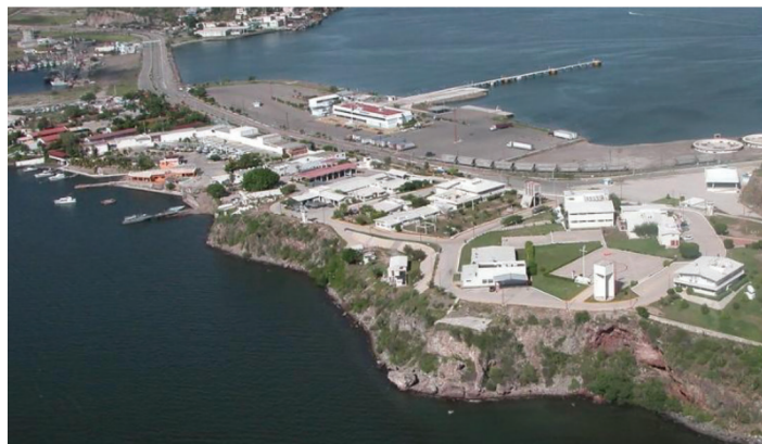
Vista Pacifico LNG project site at Topolobampo in Sinaloa
