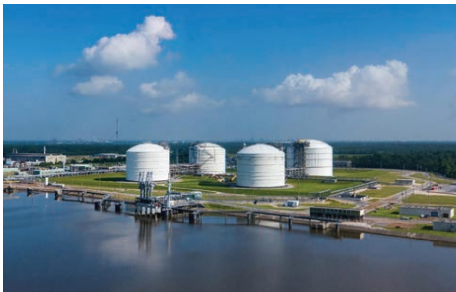
Energy Transfer's Lake Charles LNG import facility located on the Calcasieu ship channel in Lake Charles, Louisiana, US
