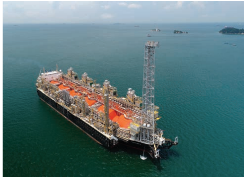
‘Golar Hilli Episeyo’ - Complete topsides design including PRICO® liquefaction on world’s first conversion FLNG, which is in continuous commercial operation since its start-up in April, 2018 without any interruption.
