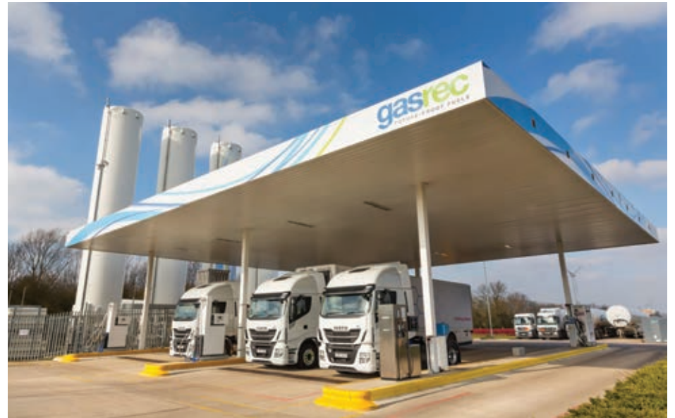
BioLNG fuelling station
