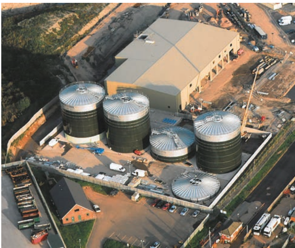
Anaerobic Digestion Plant in Staffordshire, West Midlands
