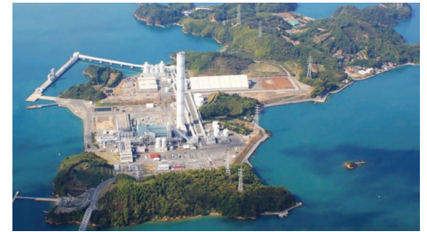
Bird's eye view of Osaki CoolGen IGCC
