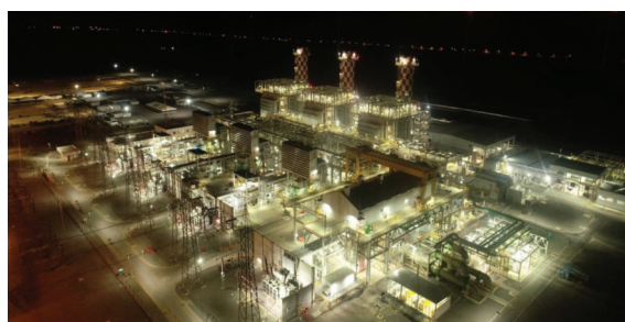
Night-time view of the 1.5 GW Port of Sergipe I Complex
