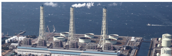
Overview of Anegasaki Thermal Power Station after new units 1 through 3 start commercial operation
