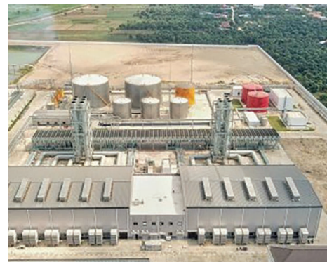
EDC's new plant consist of 11 MAN 18V51/60DF engines
