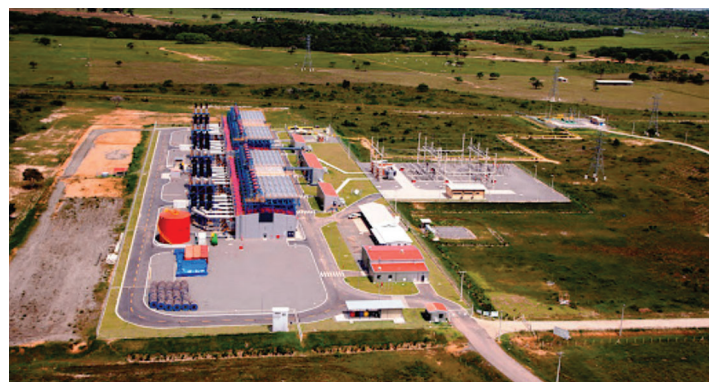
One of three emergency power units will be built next to UTE Luiz Oscar Rodrigues de Melo
