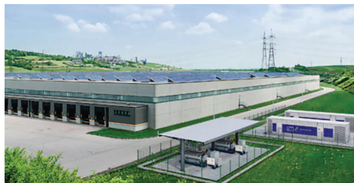
The portfolio made available through ‘Energy as a Service’ ranges from CHP units to battery containers and complex microgrids.
