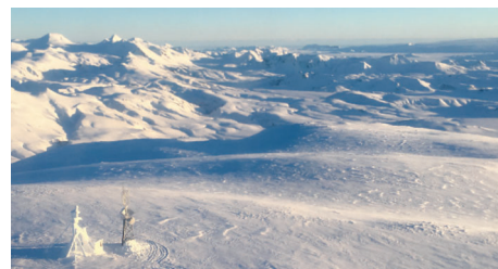
Off-grid genset installed on behalf of Neyðarlínan ohf
