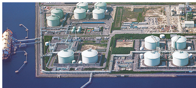
JERA's Yokkaichi LNG import terminal and power station
