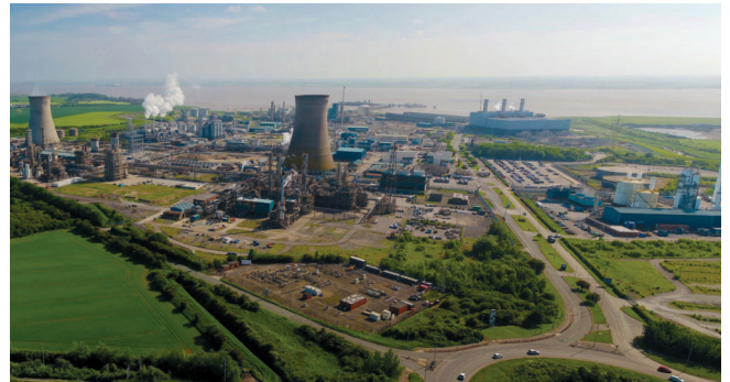
View of H2H Saltend plant, situated just east of Hull on Humber estuary.
