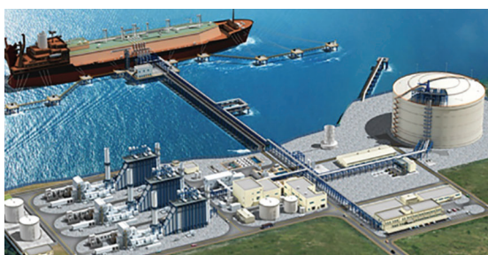
Render of AES Colón CCGT by its former owner, Inversiones Bahia
