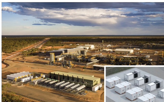
Decentral power unit, built by Zenith in Australia
