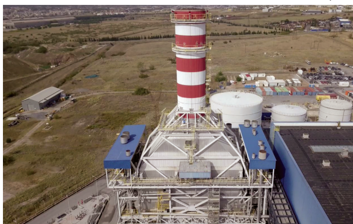
Aerial view of ELPEDISON's gas-fired power plant
