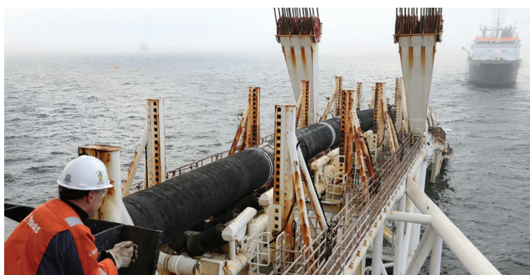
Pipe-laying for Nord Stream 2
