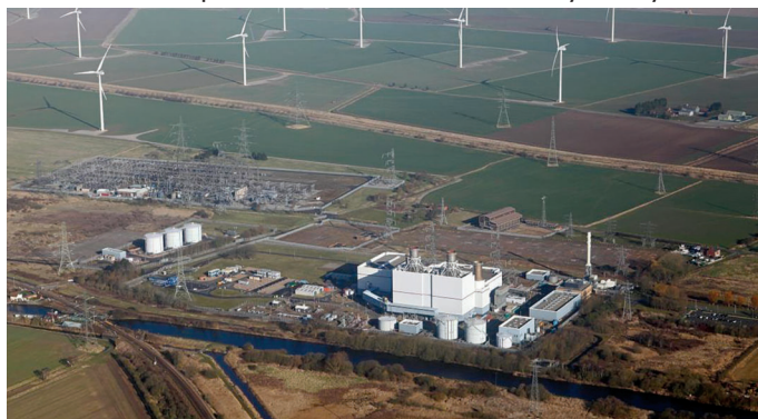
Site of SSE's Keadby Hydrogen and existing CCGTs
