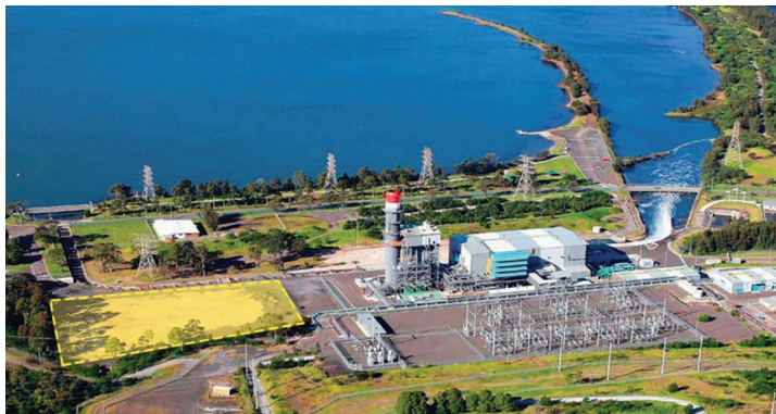
Tallawarra A power station in NSW, Australia
