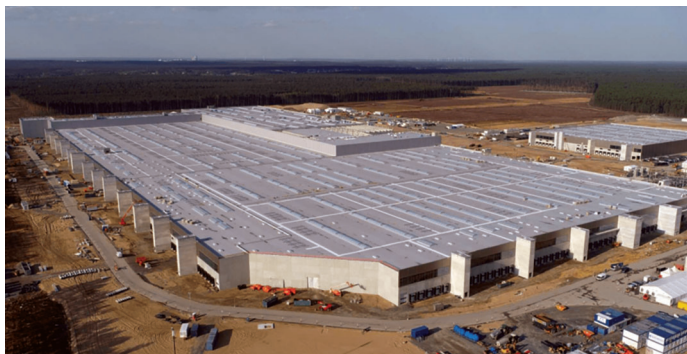
Works progress on Tesla's Gigafactory-4 at Grünheide near Berlin
