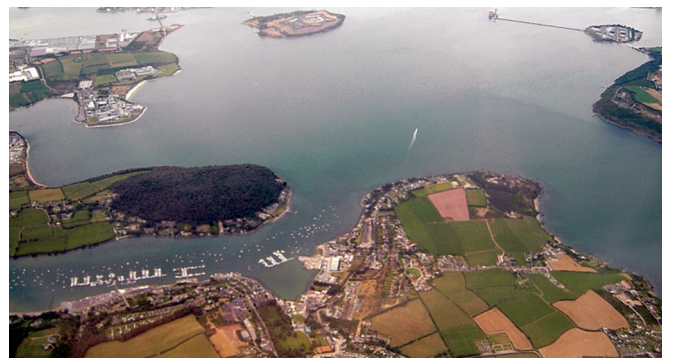
View of Lower Cork harbour, where EI-H2 will produce green hydrogen
