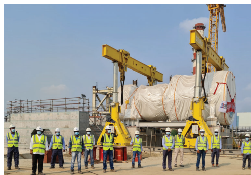
Arrival of GE 9HA.01 turbine at Meghnaghat-II
