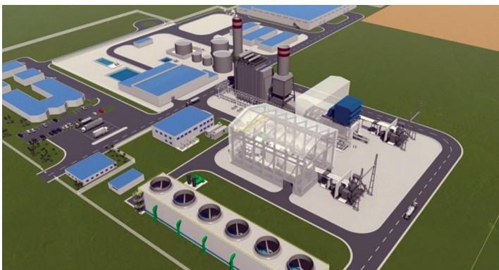
Render of Atinkou CCGT, under construction in Ivory Coast
