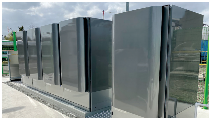
Bloom's SOFC, powered solely by hydrogen, will be used in the Ulsan pilot project
