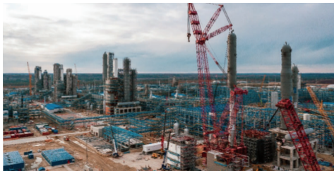
Construction of the Amur GPP which is powered by the newly commissioned Svobodny power plant.
