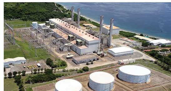
Philippine LNG will boost gas supplies to the Ilijan CCGT, under expansion
