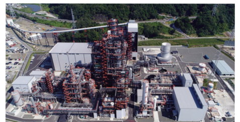
View of Nakoso IGCC plant
