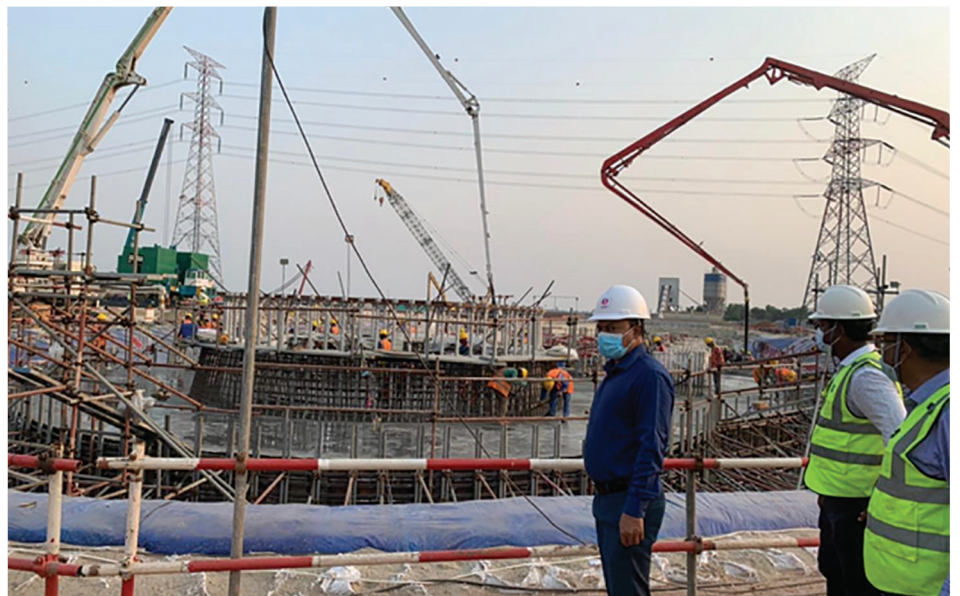
Construction site of Bangladesh Gas' rLNG-fired power plant
