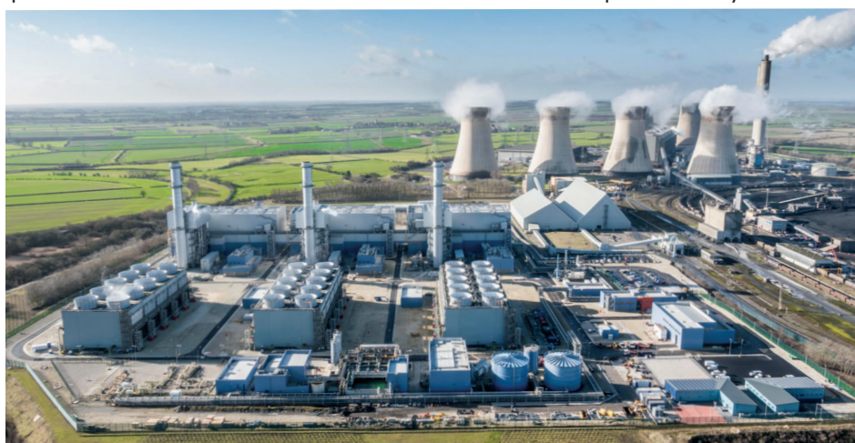
View of EDF's West Burton B combined-cycle power station
