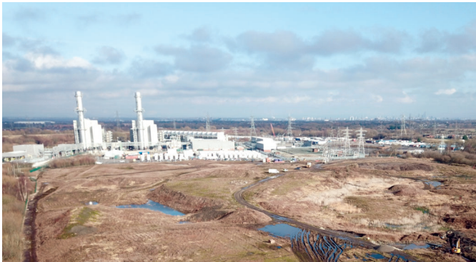
Site view of the Trafford Low Carbon Energy Park
