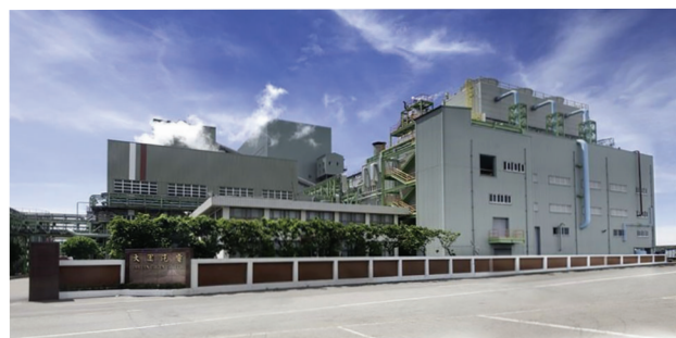
aipower's CHP in Taoyuan City will be retrofitted with dual-fuel engines
