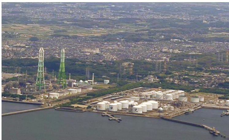
View of Chita Thermal Power Station
