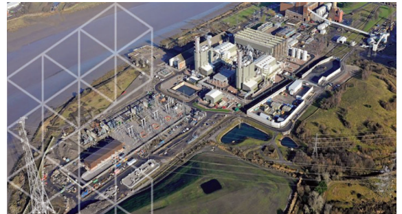
Calon Energy power station at Sutton Bridge
