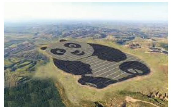
Panda-shaped 50 MW solar PV project in Datong, China.
