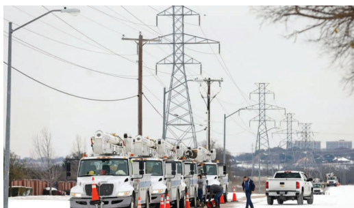
Texan power lines in the snow
