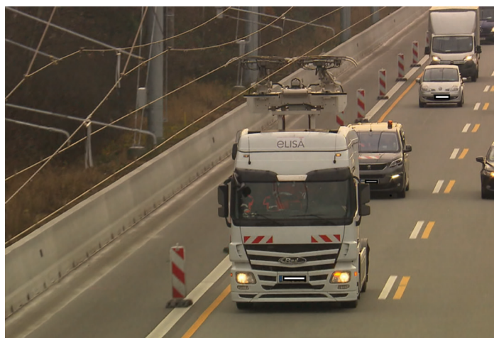
View of the so-called 'Hessen mobile' highway
