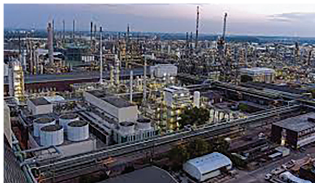
BASF's chemical production site at Ludwigshafen, Germany
