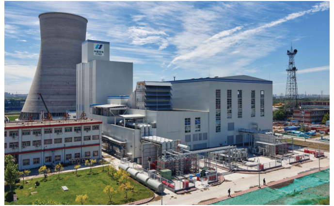
Junliangcheng CHP in Tianjin, Hebei province
