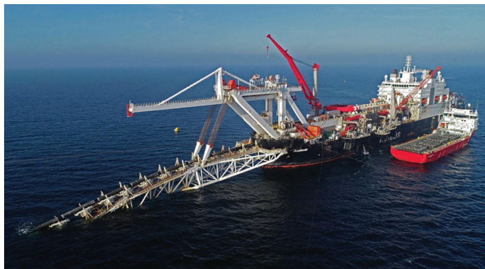
Pipe-laying vessel for Nord Stream 2
