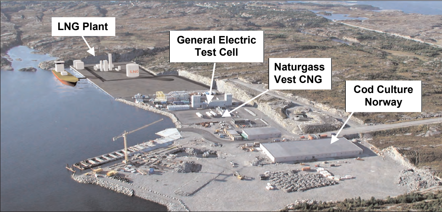
Figure 3. Appearance in 2004 of Kollsnes Industrial Park
