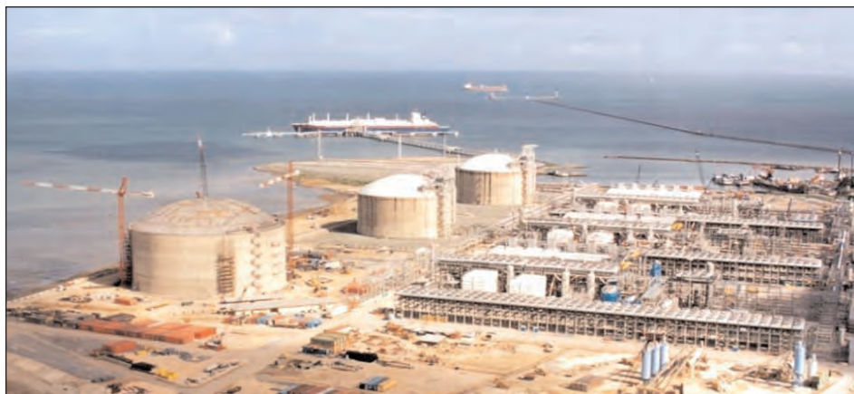
The Atlantic LNG terminal. New storage tank and trains 2 and 3 under construction (in foreground)
