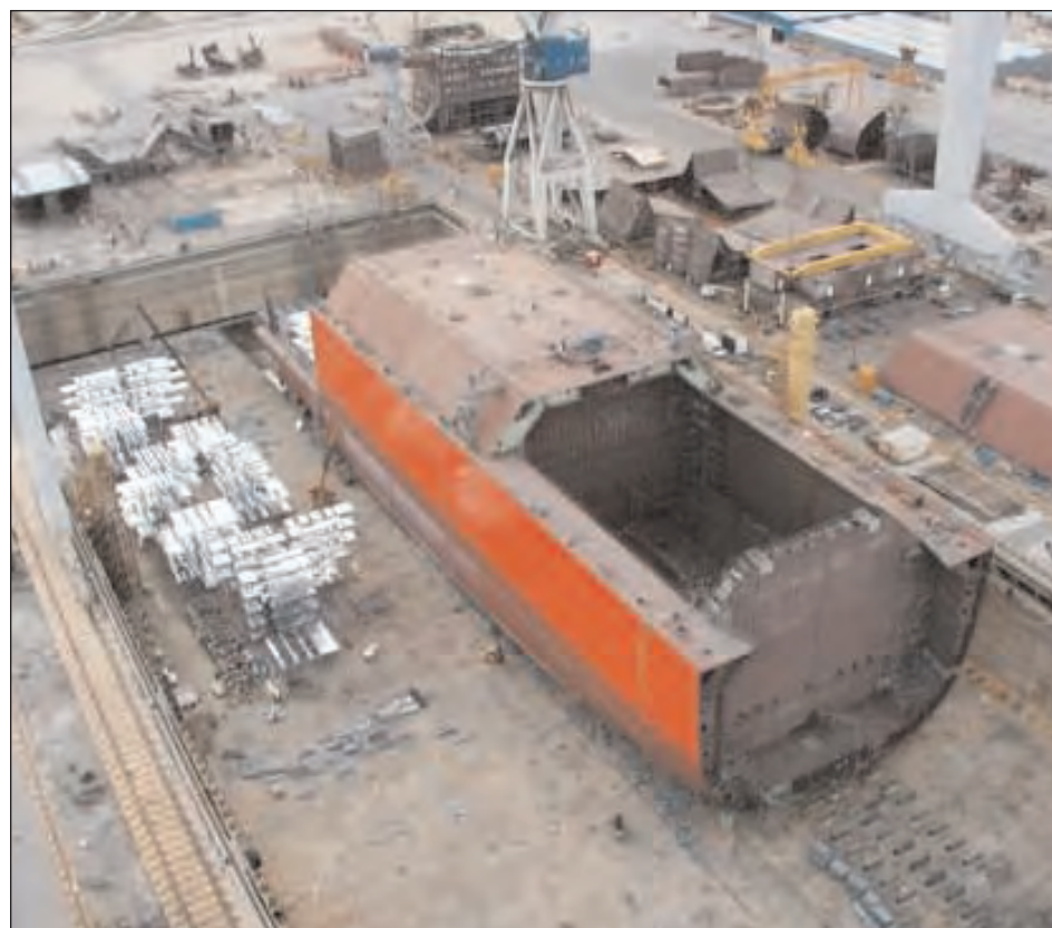
Figure 2: One of the LNG Carriers under construction for the Egypt project : Status of NB 103 for UF at IZAR - Puerto Real in June 2002
