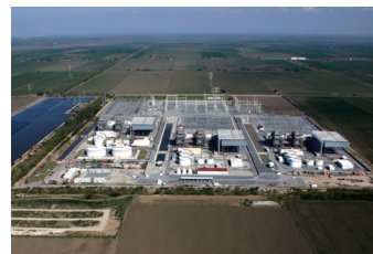
View of Rio Bravo power units II-IV
