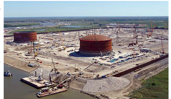
Construction works at Calcasieu Pass LNG terminal
