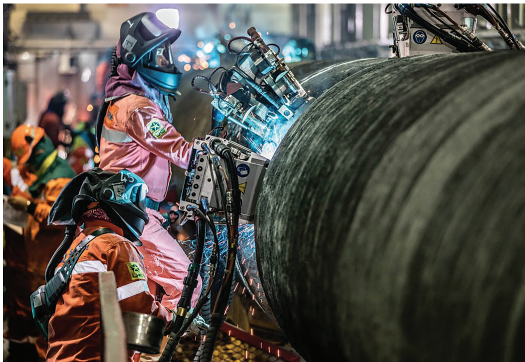
Welders connect pipe joints for Nord Stream 2
