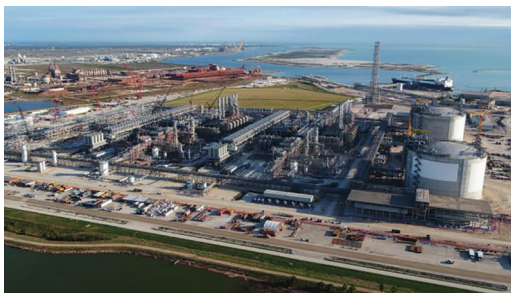
View of Cheniere's Corpus Christi LNG complex
