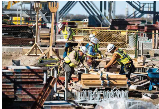
Bechtel workers at the construction site for Sabine Pass Train 6
