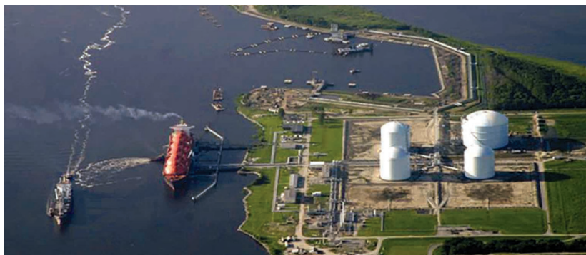
View of Southern LNG export facility in Georgia
