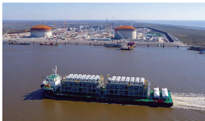
Modular construction has enabled the possibility of Calcasieu Pass starting operations early
