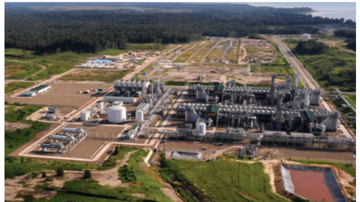
BP-operated Tangguh LNG plant in West Papua
