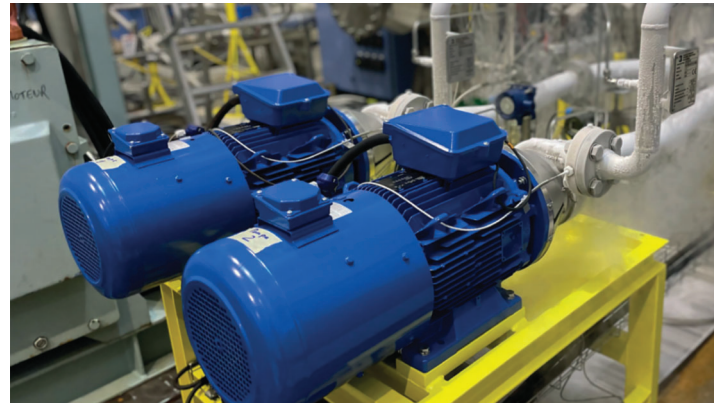
Cryostar pumps undergoing an endurance test at centre
