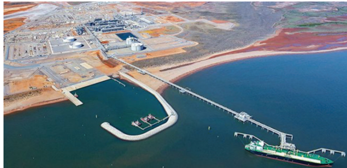
All five LNG Trains at the Pilbara plant are now operating
