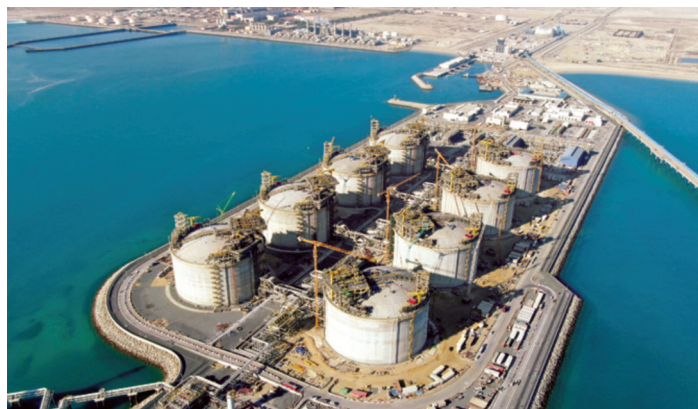
Kuwait terminal with four completed tanks and four being built in project run by Hyundai Engineering of Korea
