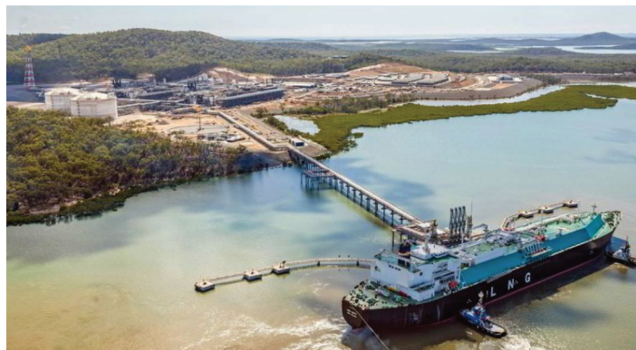
Santos-operated Gladstone plant on Curtis Island
