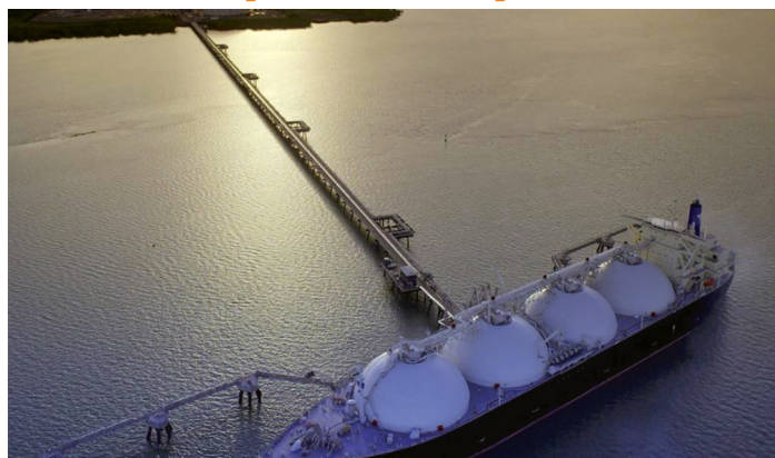
A dusk cargo lifting at Darwin LNG export plant
