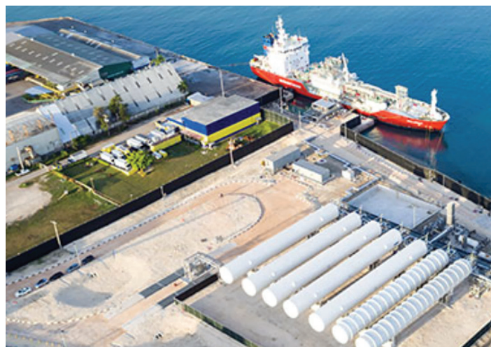
ISO containers will bring LNG to Mexico and Nicaragua
