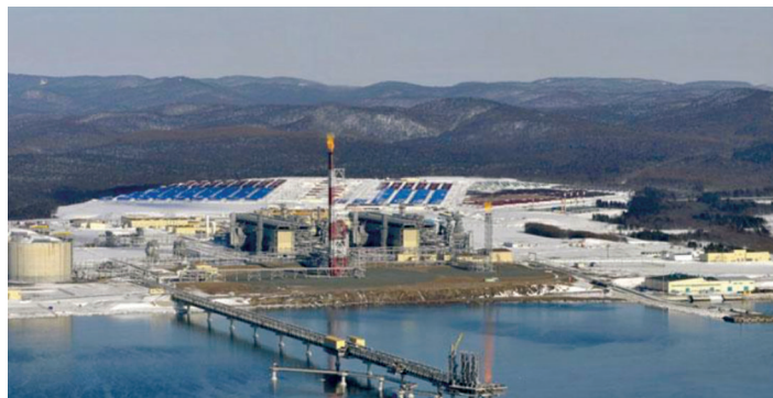
The two-Train facility at Prigorodnoye on Sakhalin Island
