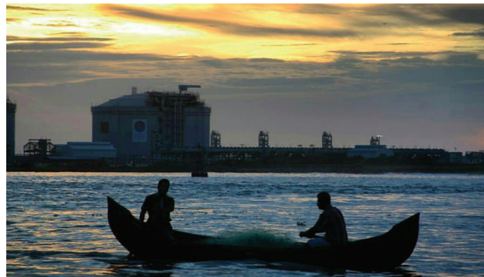
The Dahej LNG import terminal located north of Mumbai
