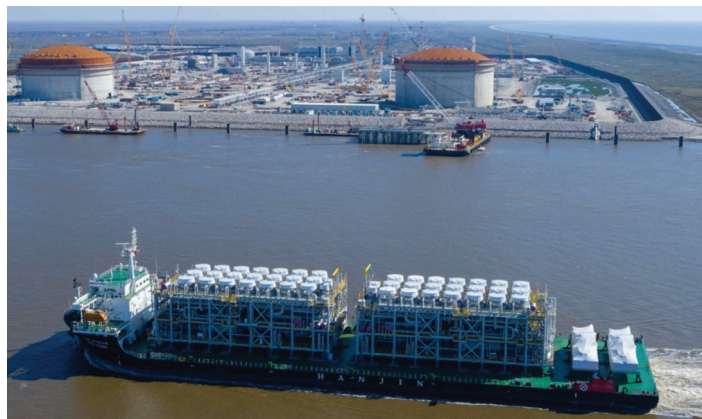
Plant is being built with delivered modular Trains
