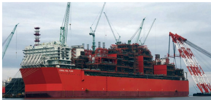
Topside modules were installed on the 'Coral-Sul FLNG' vessel at Samsung Heavy Industries in South Korea
