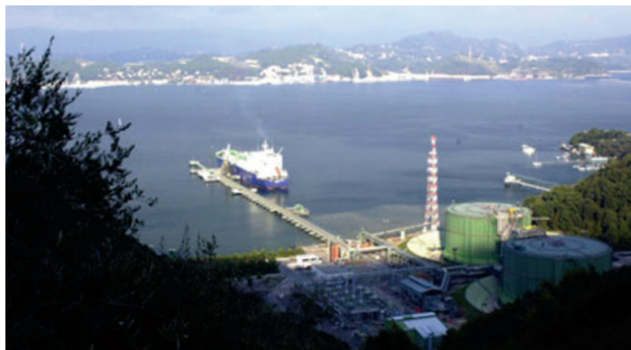
Onshore Panigaglia LNG import terminal near La Spezia
