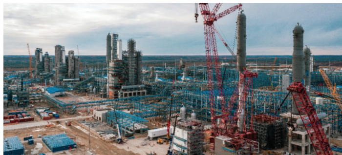
Amur Gas Processing Plant construction in Russian Far East
