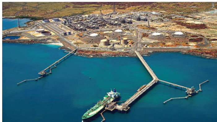
Woodside's North West Shelf plant, Australia's oldest
