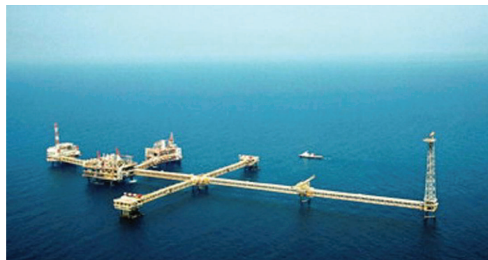
North Field project is located about 80 kilometres off the mainland of Qatar and will boost Ras Laffan supply
